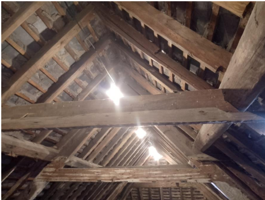
Figure 10: Overview of the internal roof structure and loft space.
