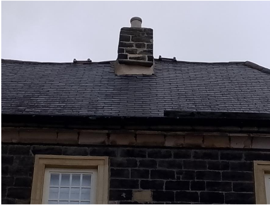
Figure 5: Close-up of the roof tiles and chimney.
