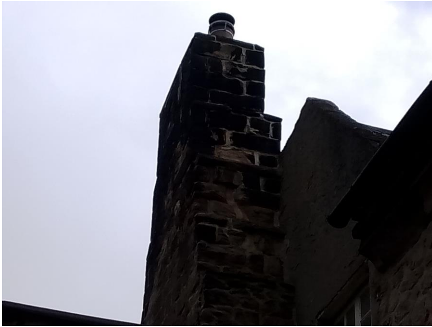
Figure 7: Close up of the chimney.
