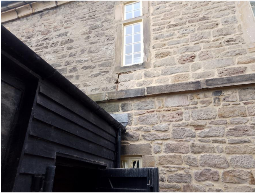
Figure 9: View of external stone walls.
