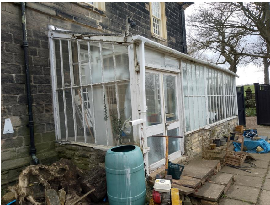
Figure 8: View of the glass section at the rear.
