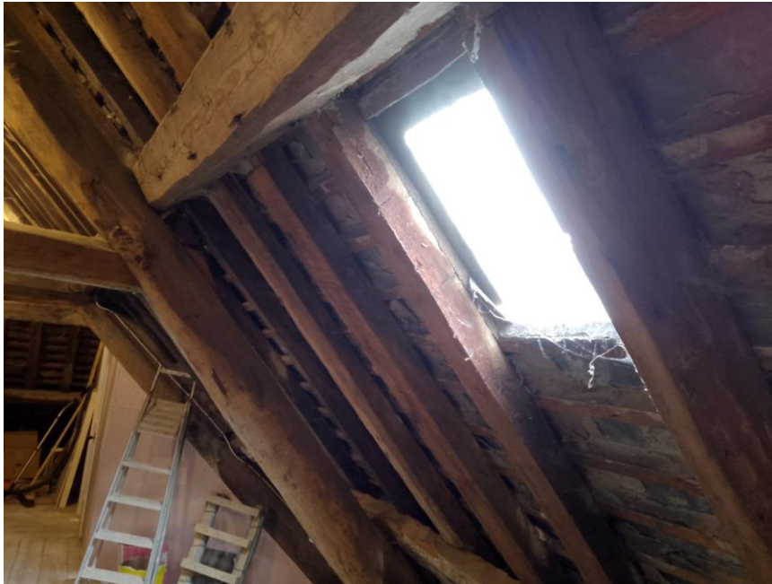
Figure 1: View showing light coming into the loft space from the outside.
