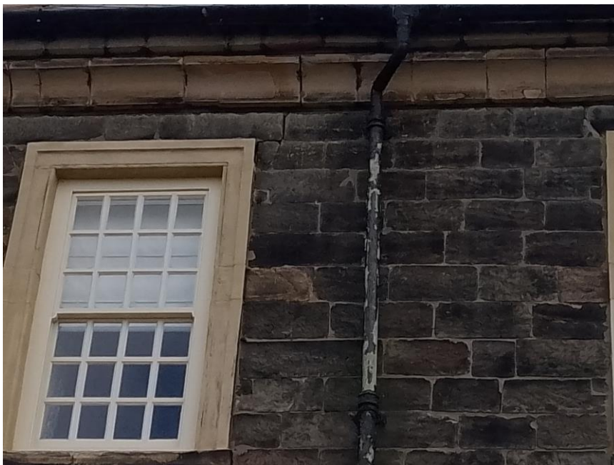
Figure 6: External walls with crevices suitable for bats.
